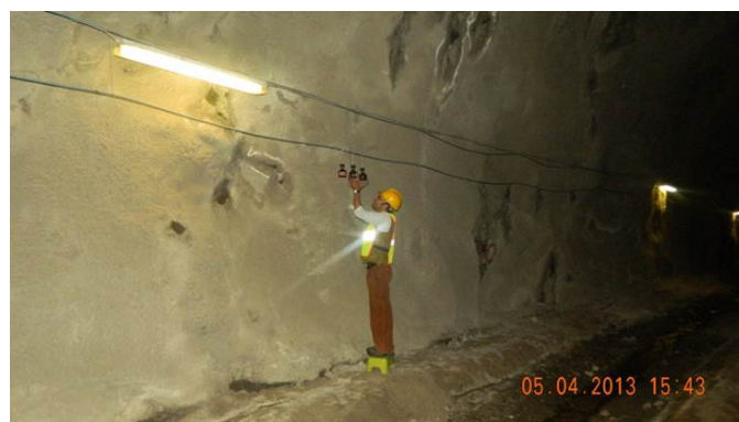
FIGURE 2. Electrets mounted in groups of 3 on the walls of the tunnel close to the vehicle cross-cuts. During the excavation period (1973 - 1984) the composition of the mountain range mainly composes of
