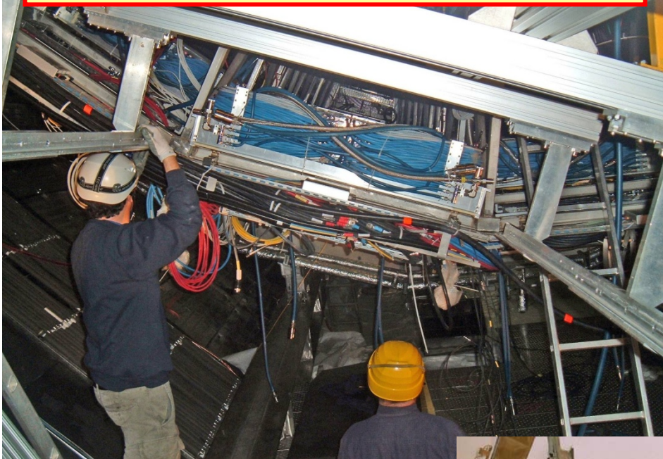
Insertion of final TOF super module
